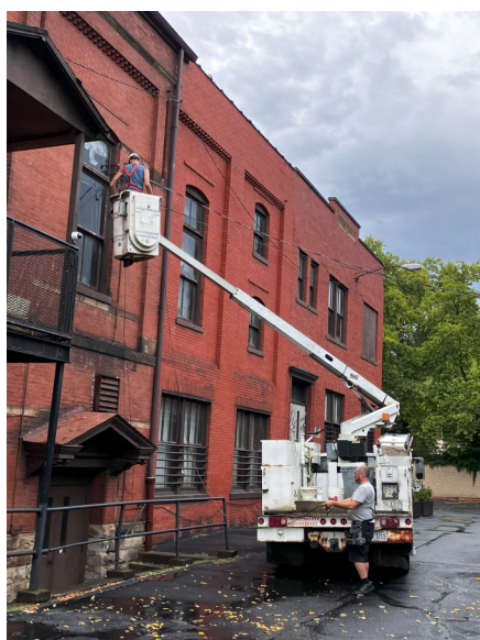
Rick Smetana and Chuck Shieff installing cameras for the security system
